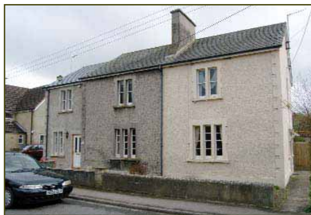
Figure 12. Estate cottages – south side of Salisbury Road
