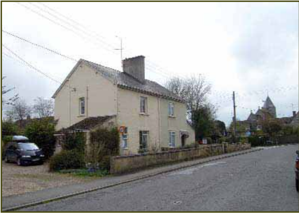
Figure 19. Nos. 14 & 16 Salisbury Road – note loss of rendered mullions and timber sashes.
