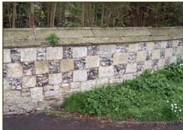
Figure 14. Superior quality and materials of boundary wall to Montrose House.
