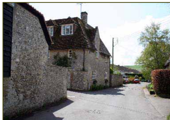
Figure 8. Duck Street – important group framing views out to the valley
