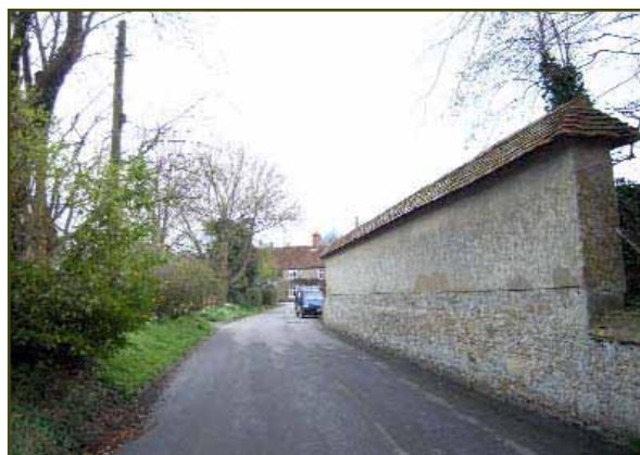
Figure 15. Cob and stone boundary wall on a grand scale, Montrose House
