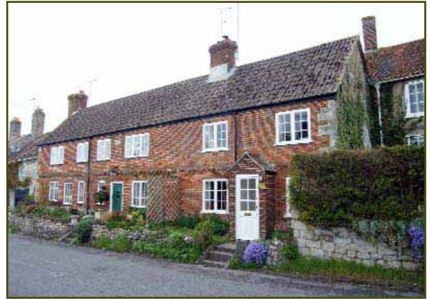
Figure 4. Nos. 15/ 17 Salisbury Road – distinctive use of brick and a double Roman interlocking tile
