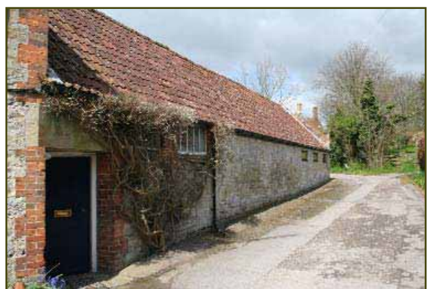
Figure 10. Outhouses to the Malthouse
