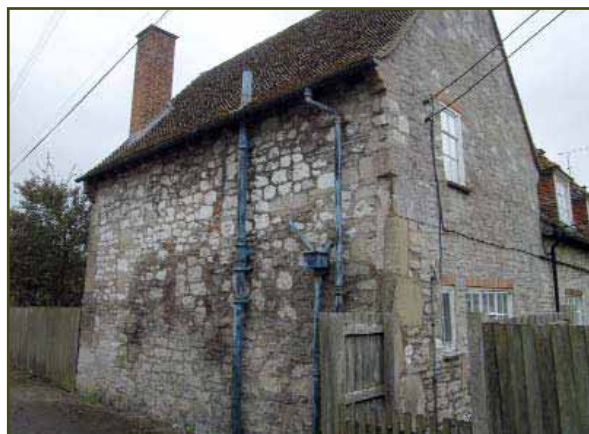
Figure 16. North (roadside) elevation to No.1 Church Cottages, Duck Street.
