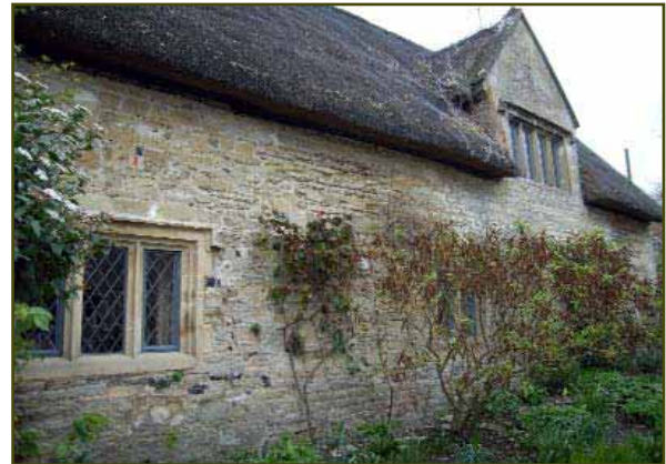
Figure 17. 'Mean' layer of combed wheat reed thatch; Greystones Cottage, Duck Street
