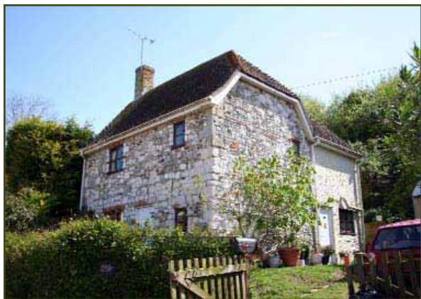
Figure 6. Berwick Lane – use of chalk blocks from the adjacent former chalk pit
