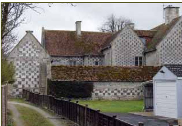
Figure 9. Stone and flint chequerwork; Montrose House (former Rectory)
